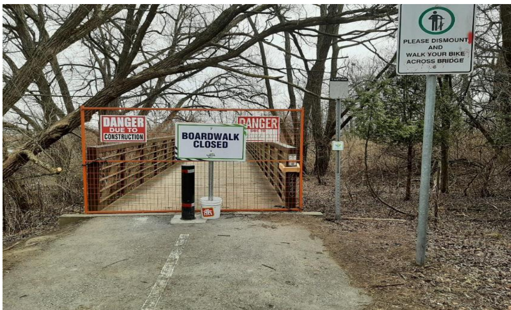
Fig 1. West Side Duffins Creek Bridge
