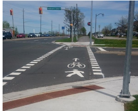
Seaboard Gate - in Place
