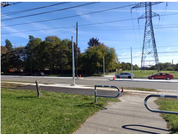
Crossing Under Construction at Manning Rd.
