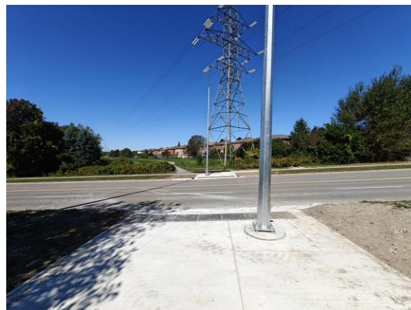
Crossing Under Construction at Rossland Rd.
