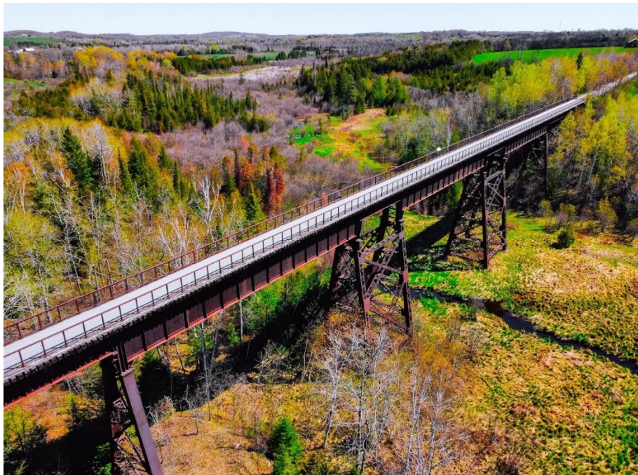
Doube's Trestle Bridge
