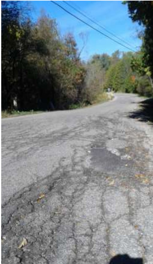
Greenwood Rd. - Surface Deterioration Forced to ride in centre of road with blind corners
